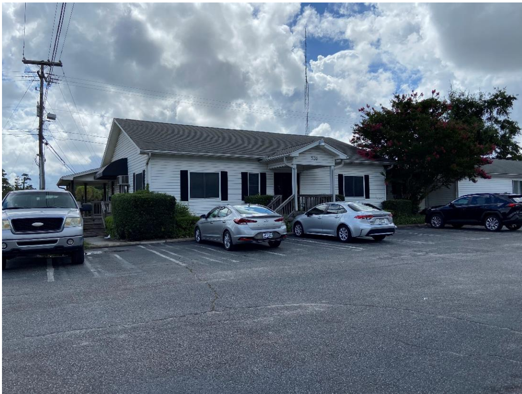
Photo #6 – Wando Trucking (510 Wando Lane) : Office buildings facing northeast.
