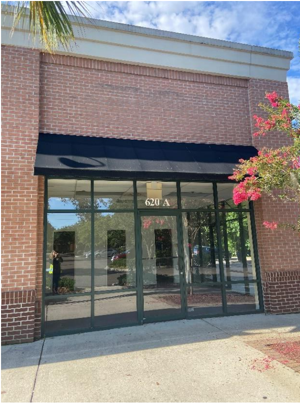
Photo #3 – Lyerly's Cleaners (620 Long Point Road) : Vacant suite, former location of Lyerly's.
