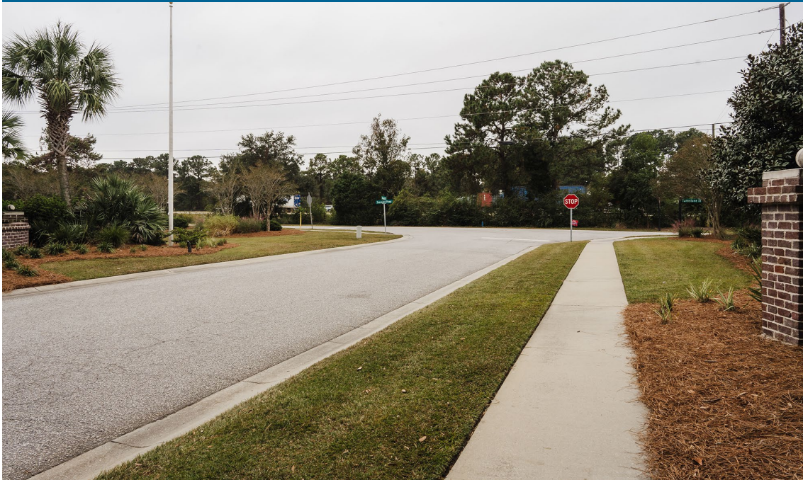
Existing conditions at Seacoast Parkway and Shoals Drive
