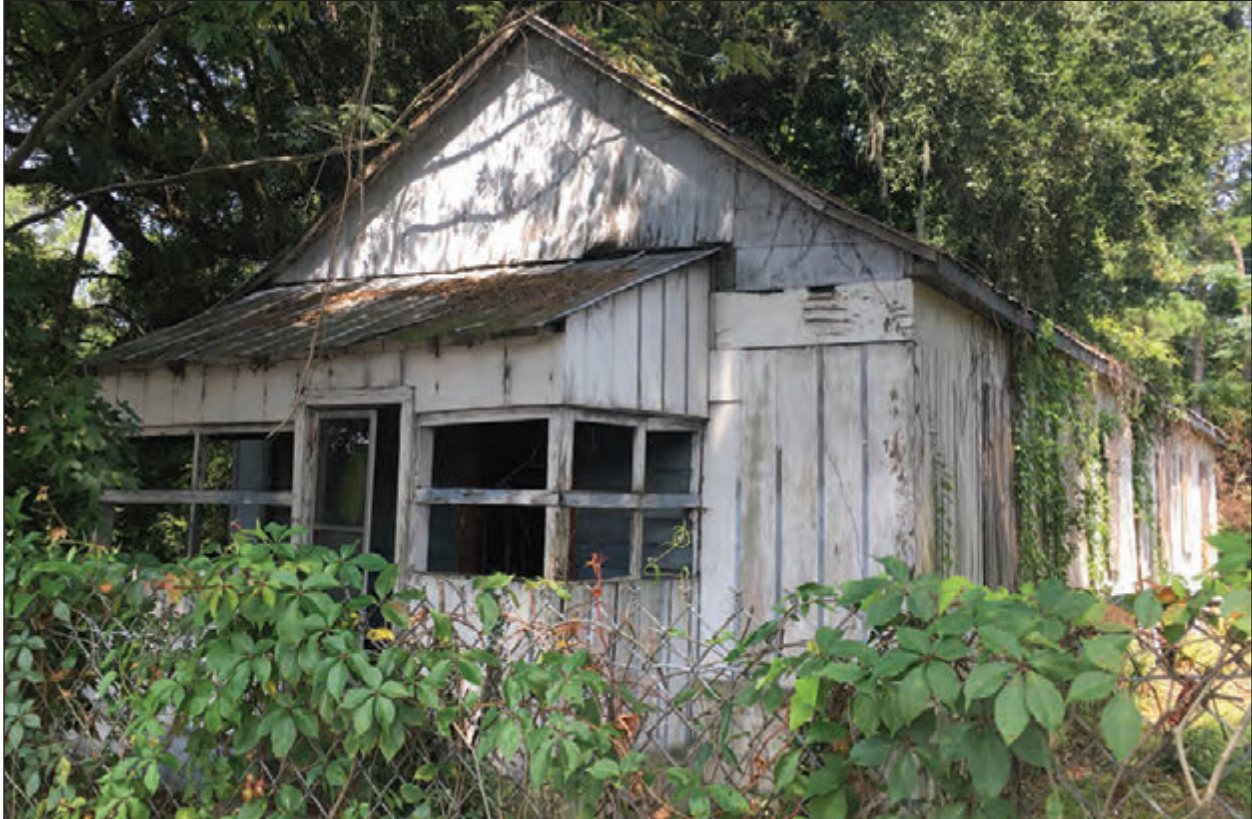
Figure 5.11 SHPO Site No. 7802 on CCP 5560000312 in 2018 facing north.
