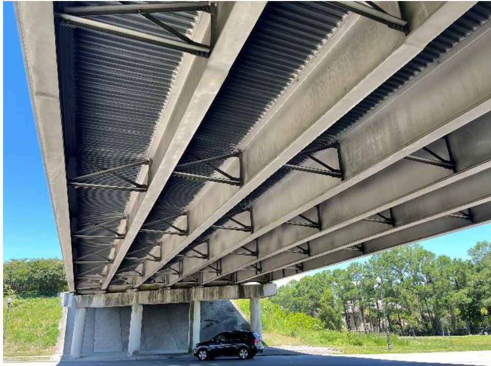
Photograph 14: Underside of the I-526 bridge over Long Point Road
