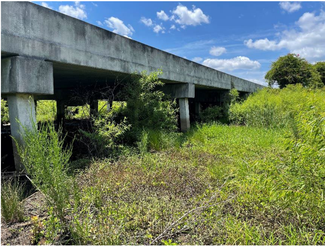
Photograph 5: Palustrine emergent wetland between I-526 and Chimney Bluff Drive
